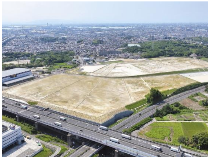
Obu Tokai Industrial Park Development Project (229,351 square meters)
